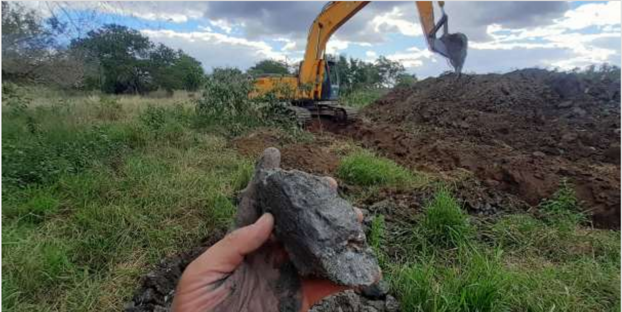
Figure 9.2 Trenches were planned based upon historical data and surface trends observed (Source: QP).
